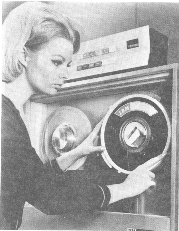
Figure 7-30. IBM 2420 Magnetic Tape Unit Model 7 with Wraparound Cartridge
